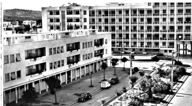
Figure 8: Public garden within a large-scale development project, Menzah 1, 1960. Source: Gharbi S., 2023.
