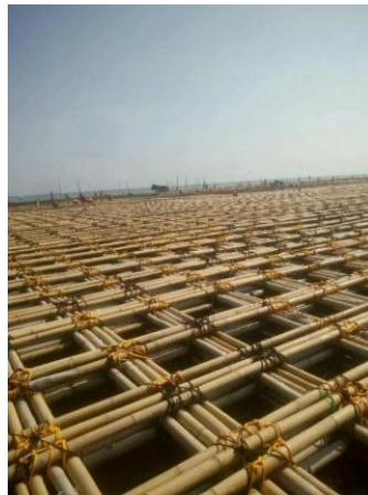
Figure 1. Bamboo Mat Construction
