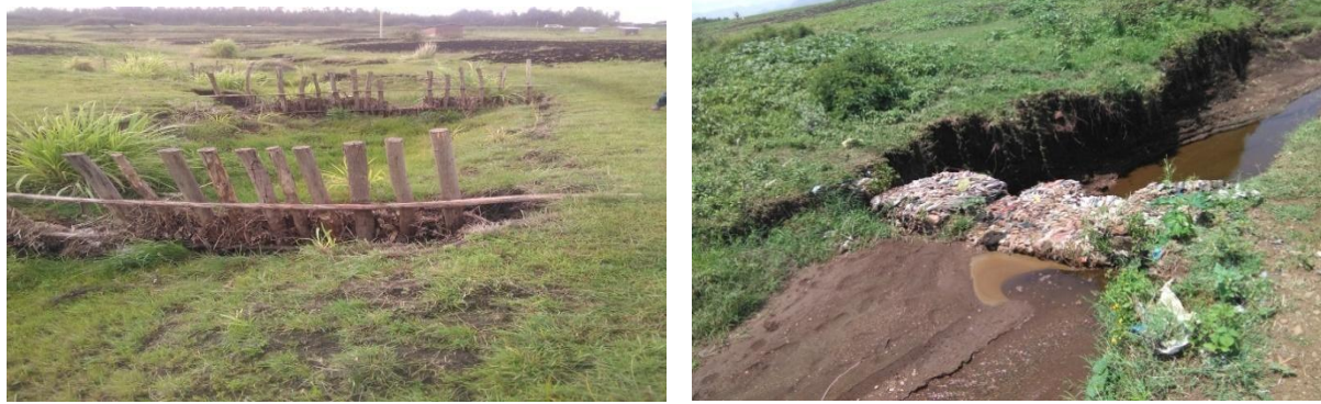
Figure 6. Check dams constructed from woods and gabions in North Gondar Zone Photo by the authors (2017).
